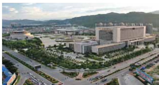
Bird's-eye view of Longyan Administrative Service Center (at the People's Square)
