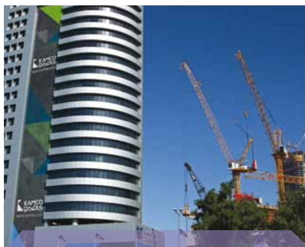
Kuwait City: skyscraper under construction.
